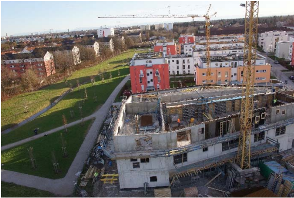
Figure 2: Aerial view of a construction site from an UAV
